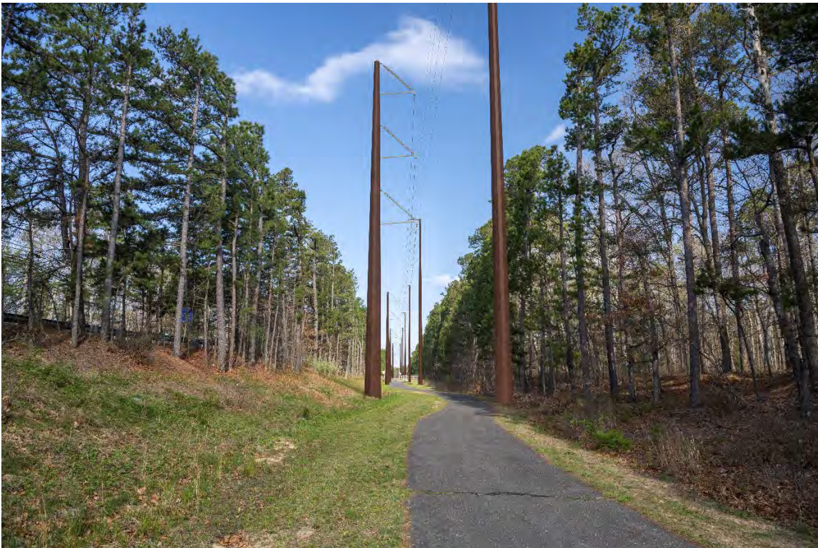
Figure 6-37. Example of Weathered Steel Monopoles along a Trail
