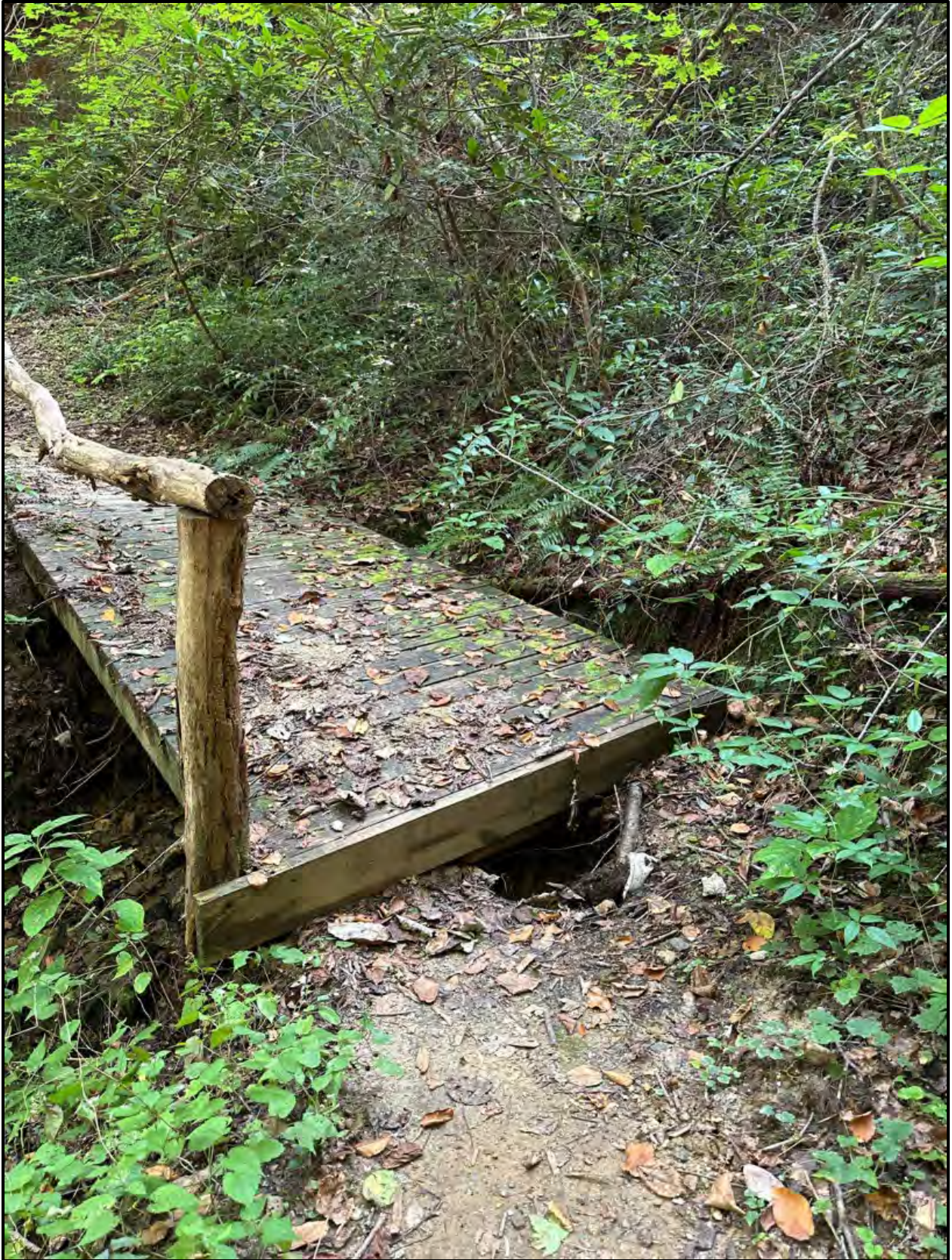
Photo 30. Trail Issue #30 - Foothills Trail, Erosion, Gully (see Figure 4.8)
