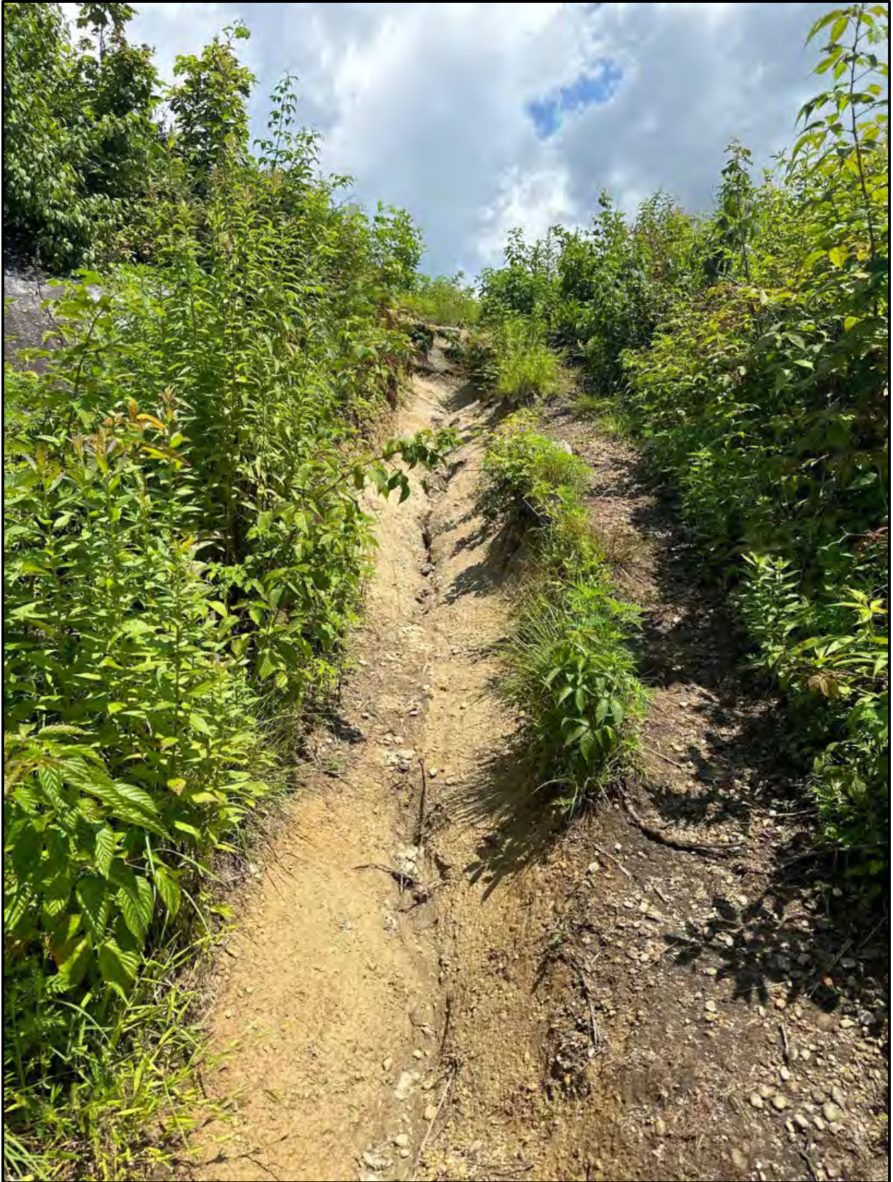
Photo 76. Trail Issue #76 - Foothills Trail, Erosion/Gully (see Figure 4.18)
