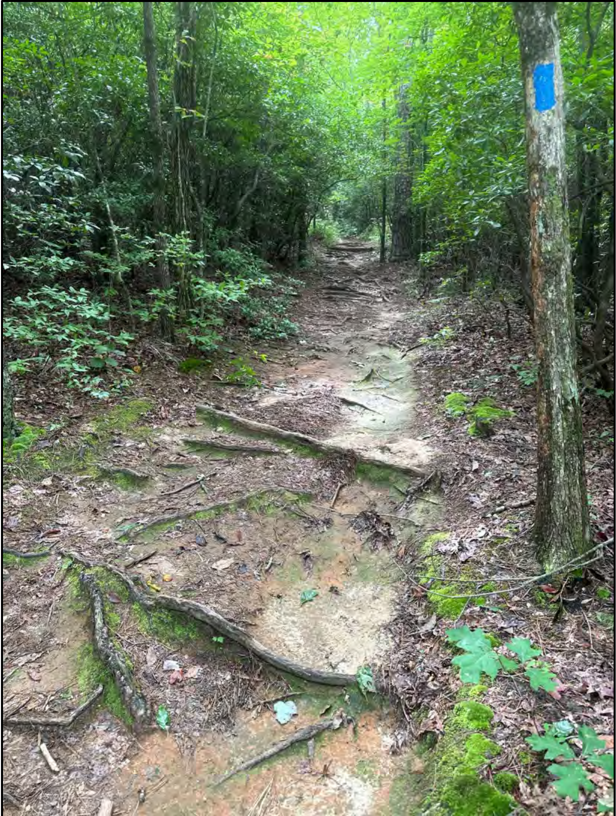
Photo 12a. Trail Issue #12 - Lower Whitewater Falls Spur, Washout (see Figure 4.4)
