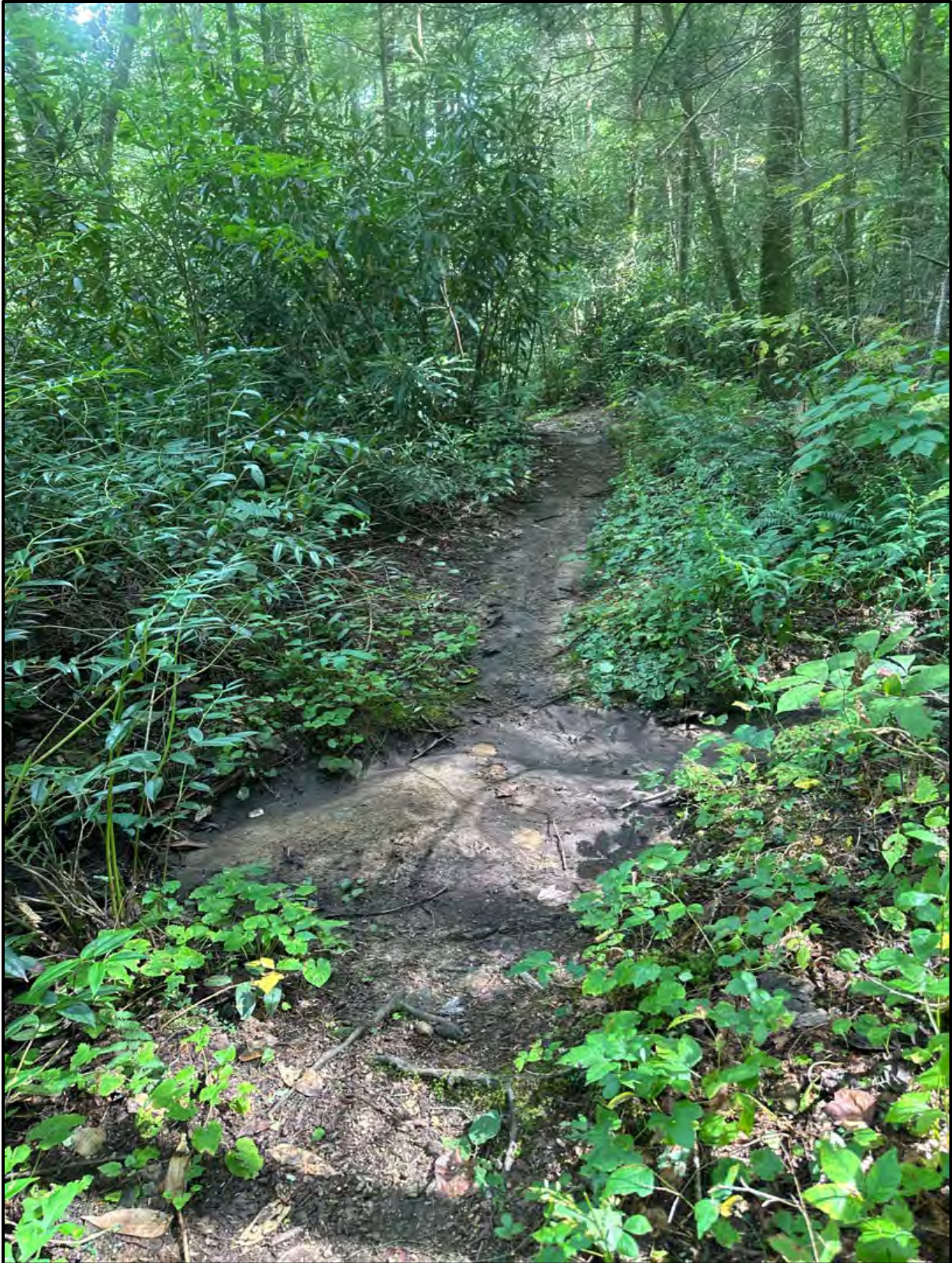
Photo 11. Trail Issue #11 - Coon Branch, Erosion, Gully (see Figure 4.3)
