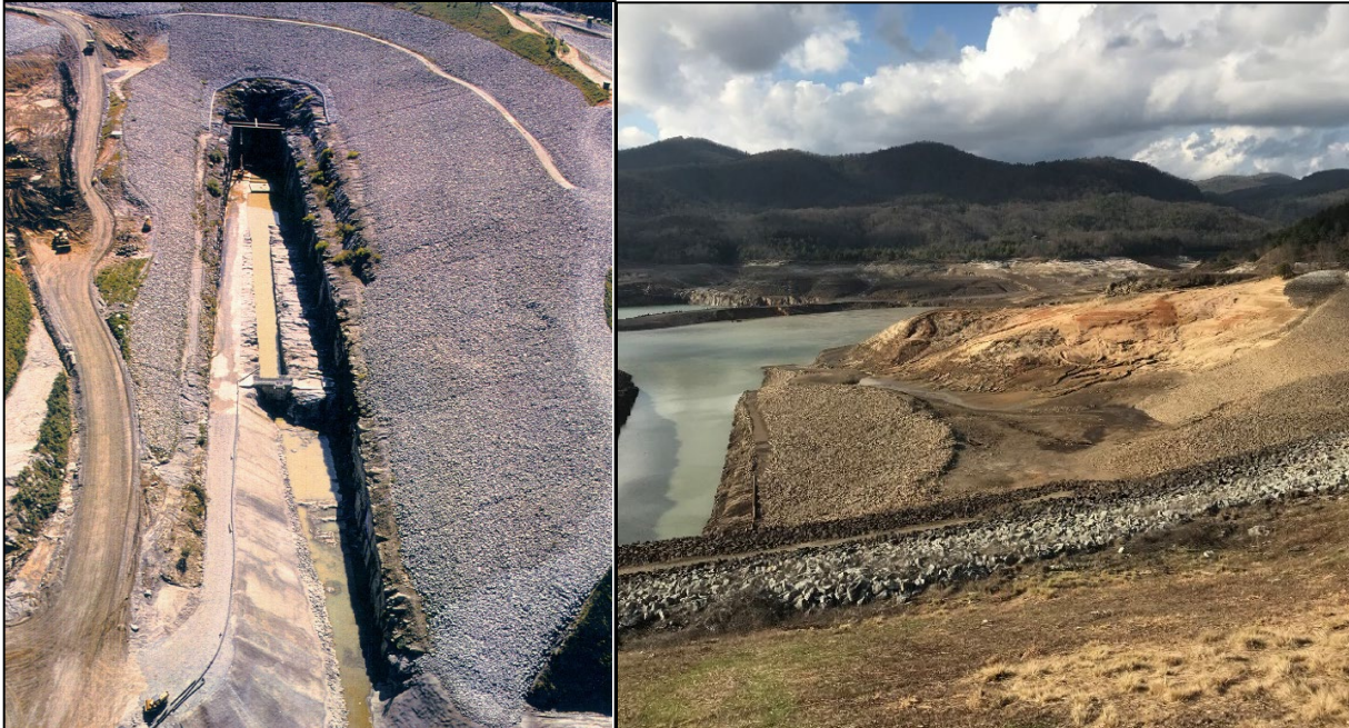
Figure A-5. Upper Reservoir Intake Channel; (left) Prior to Initial Reservoir Fill and (right) Under Full Reservoir Drawdown Condition
